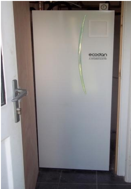
The 200 litre stainless steel cylinder comes pre-wired and pre-plumbed for ease of installation.
