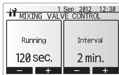
Mixing valve setting screen
