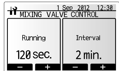
Mixing valve setting screen
