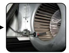
If the air curtain is going to be operated under Room Air Temperature Control it does not matter where the air temperature sensor (marked red) is located as air temperature sensing is now done at the PAR-30MAA Remote Controller. The PAR-30MAA Remote Controller will need to be set up via its Installer Menu so that temperature sensing is done at the controller. See instructions that come with the controller. Check that the dip switches on the Interface PCB are set as follows:
