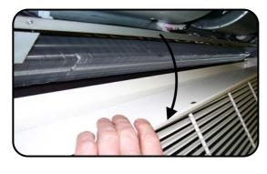
The drain tray now hinges down along its front edge and the inside surface of the tray can be cleaned. Remove all debris and deposits from the coil face, drain tray, outlet pipe, condensate hoses and the condensate disposal system. Check there are no kinks in condensate hoses. If the condensate pump is a peristaltic type change the rubber pump head tube. Refit drain tray opposite to removal.
