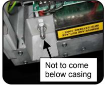
There are two M10 hanging rods at each end of the unit (four in total) that enter the casing from the top and attach to fixing brackets near the bottom of the unit (see picture above – looking up into the air curtain). Use M10 lock-nuts either side of the fixing bracket to secure the hanging rod. Do not let these four hanging rods come below the bottom of the unit casing or they may prevent the recessed grille fitting properly.
